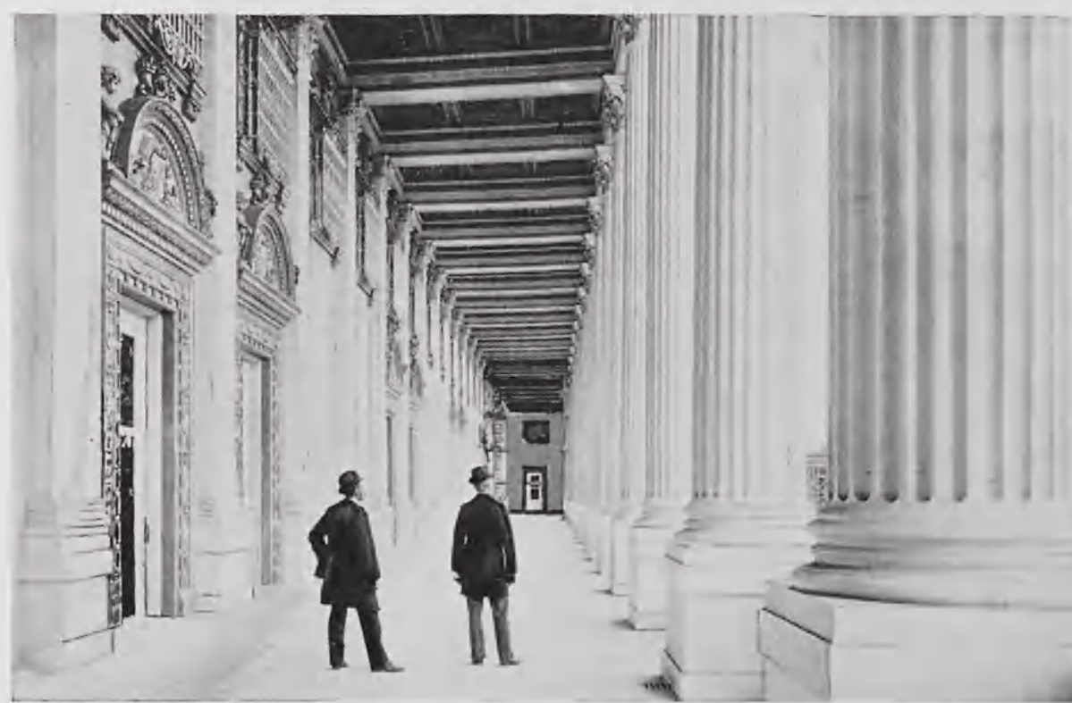
THE LOGGIA, MACHINERY HALL
